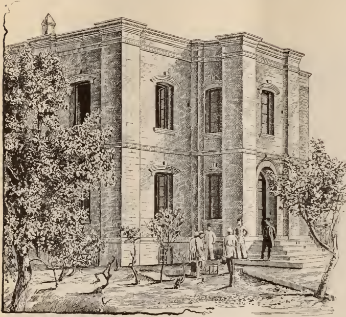
CONTAINS A CHAPEL AND SEVEN RECITATION ROOMS. BUILT IN 1891, OF RED BRICK
